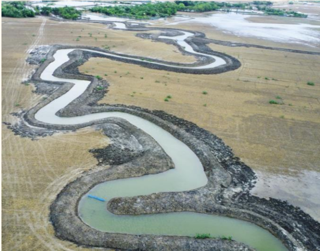
Canal Excavation to regain Fresh Water Flow
