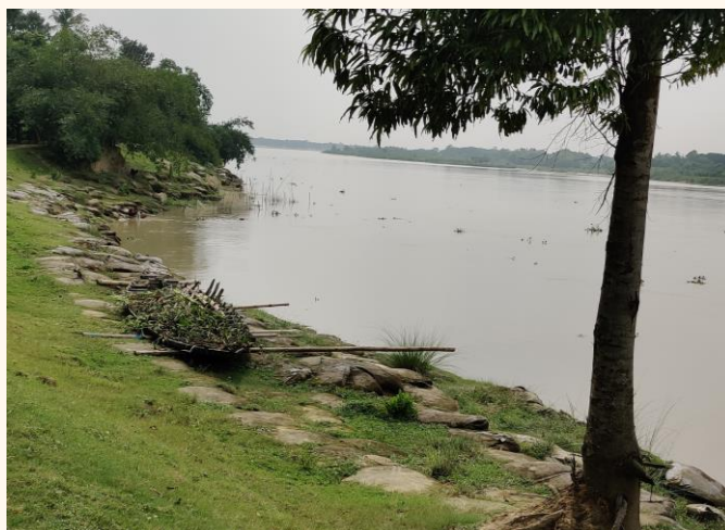
Riverbank Protection using sandbags
