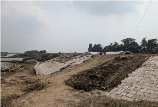
Submersible Road Construction in Flash Flood Region
