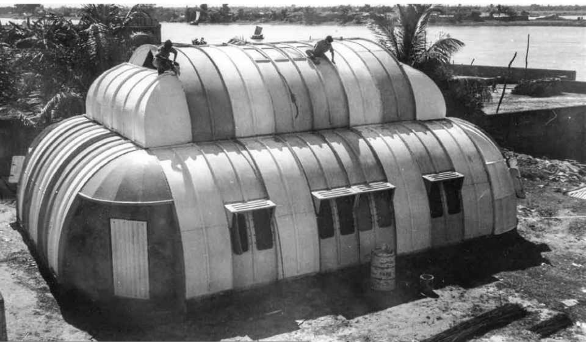
A newly-built CARE building, part of their Experimental Housing Project in Bangladesh in 1973.
