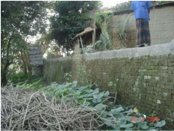
Mound protection wall in Derai
