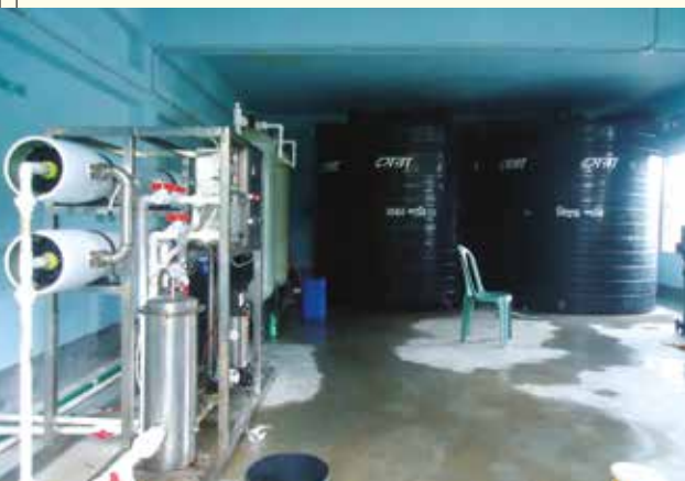
Reverse osmosis is gradually becoming a solution for drinking water in the SWR
