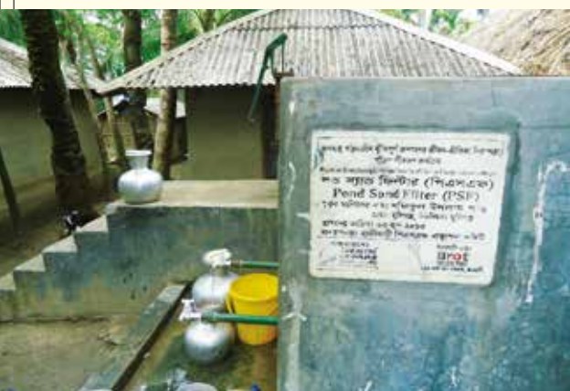
Pond-sand filter is a low-cost technology that provides for non-saline water in the SWR
